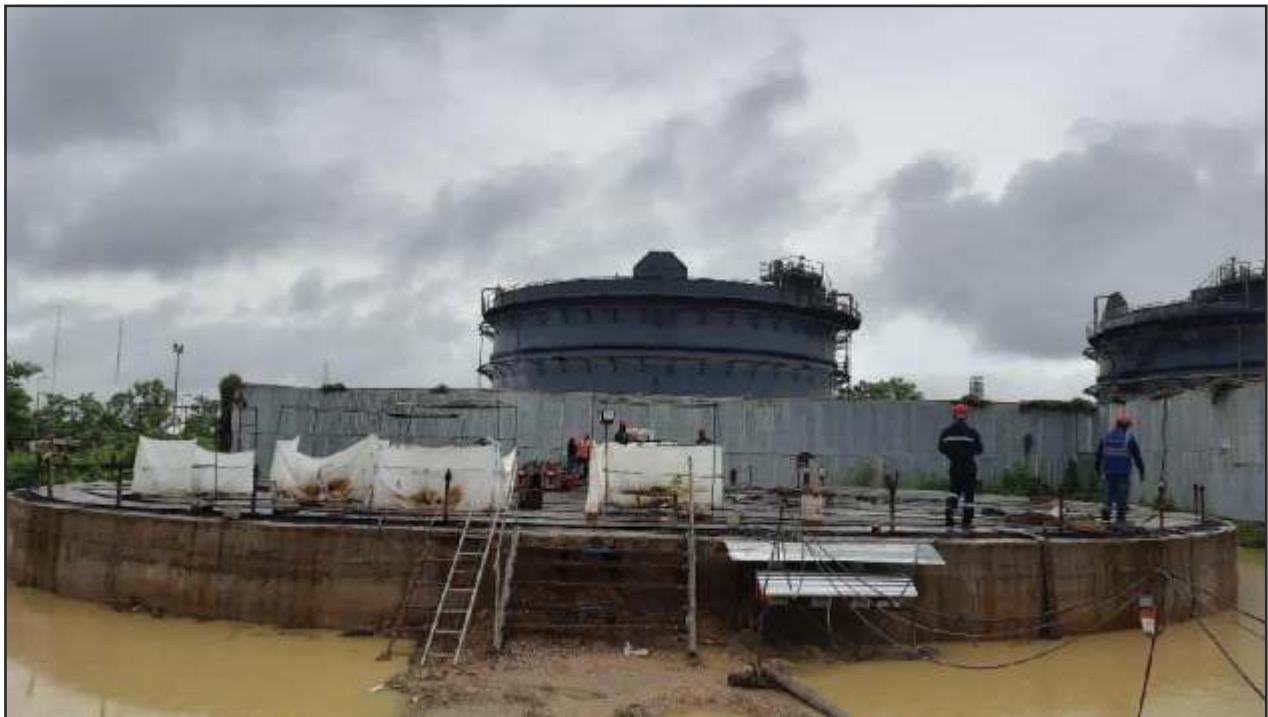
Butene-1: Structural Erection in progress in TS-5 and TS-1 Tankage Works: HDPE sheet laying completed in HPG-2
