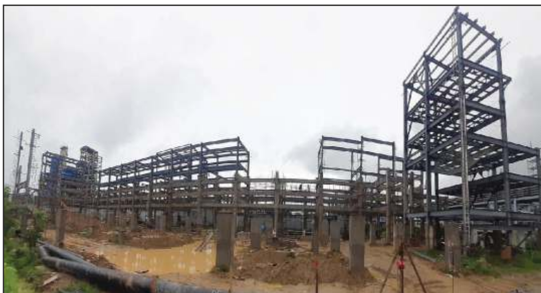
Butene-1 (Panoramic View): Structural Steel Works in progress
