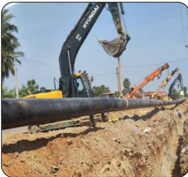
Lowering in Progress
