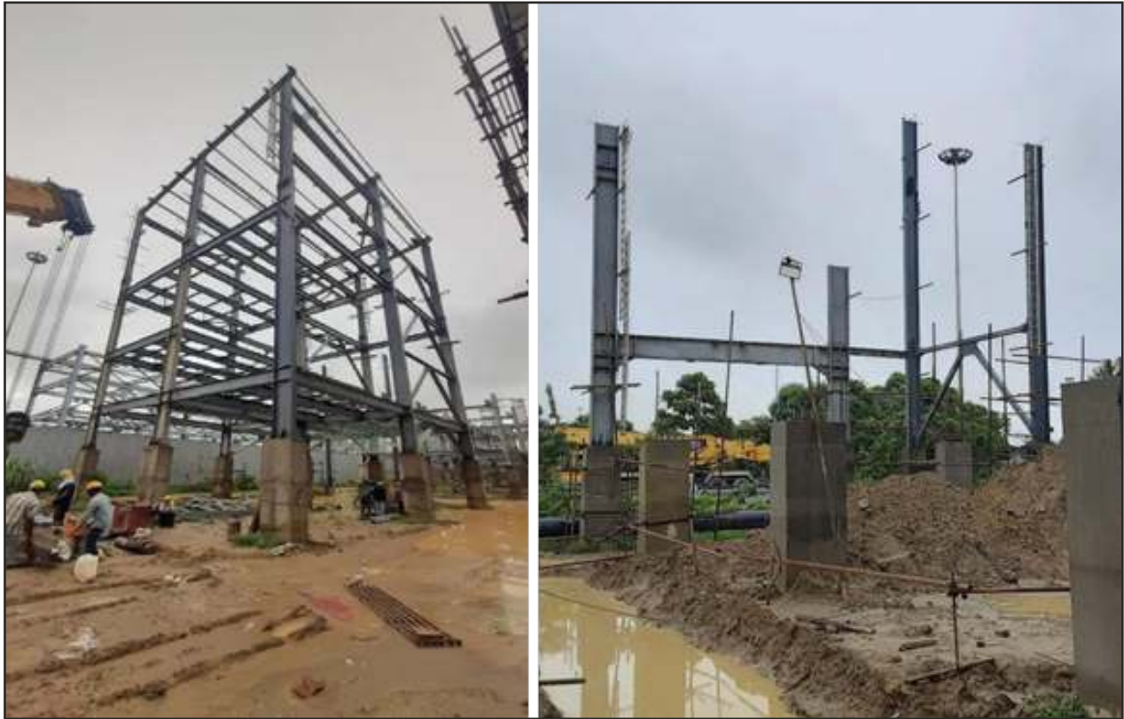
Butene-1: Structural Erection in progress in TS-5 and TS-1 Tankage Works: HDPE sheet laying completed in HPG-2
